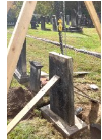
Images left to right: Staymat prepared to reset sunken and tipped stones. Epoxy and clamps are used to repair a stone, and a hoist puts it back in place.
